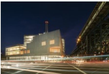
The Forum was recognized with a 2019 MASTerworks Award from the Municipal Art Society of New York, its second prestigious recognition in the architecture community. (Photo: ©Nic Lehoux)
