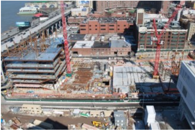
Columbia Business School site, looking north
