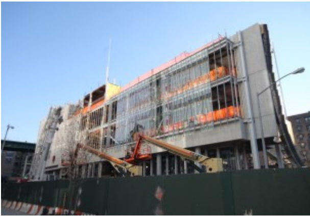
Glass façade installation on the north side of the Forum
