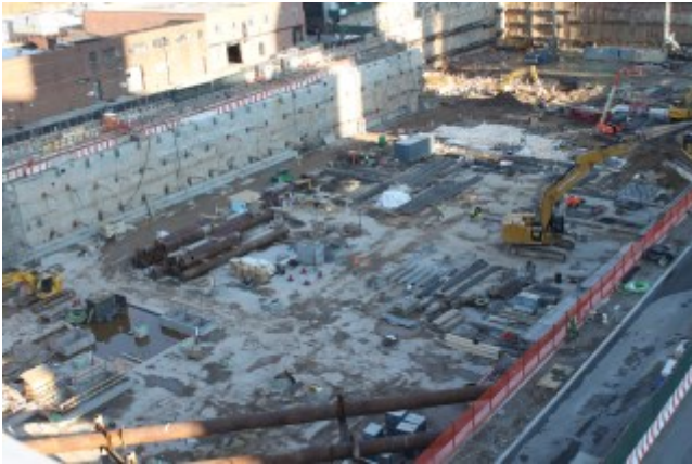
Phase 2 foundations site, looking northwest
