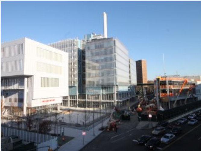
(From L to R): Lenfest Center for the Arts, Jerome L. Greene Science Center, and the Forum (under construction)
