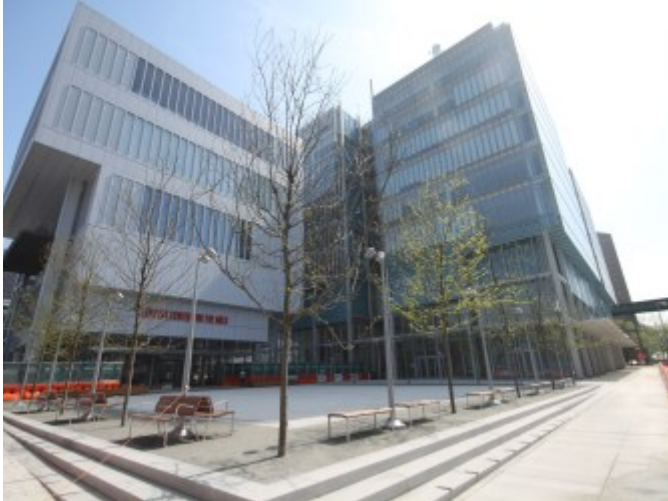
The Lenfest Center of the Arts (left) and Jerome L. Greene Science Center (right), with the Small Square in the foreground, looking northeast
