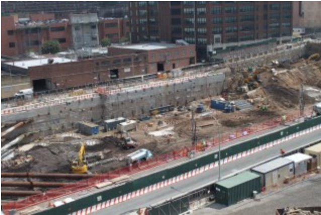
Phase 2 foundations site, looking northeast
